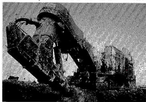
Fig 12.4 Rock breaking equipment used on site
