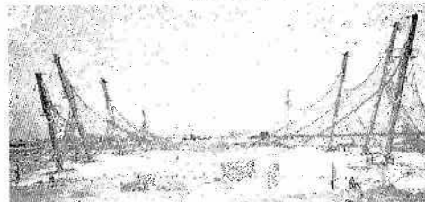
Fig 4.2 Erection of cable net on site
