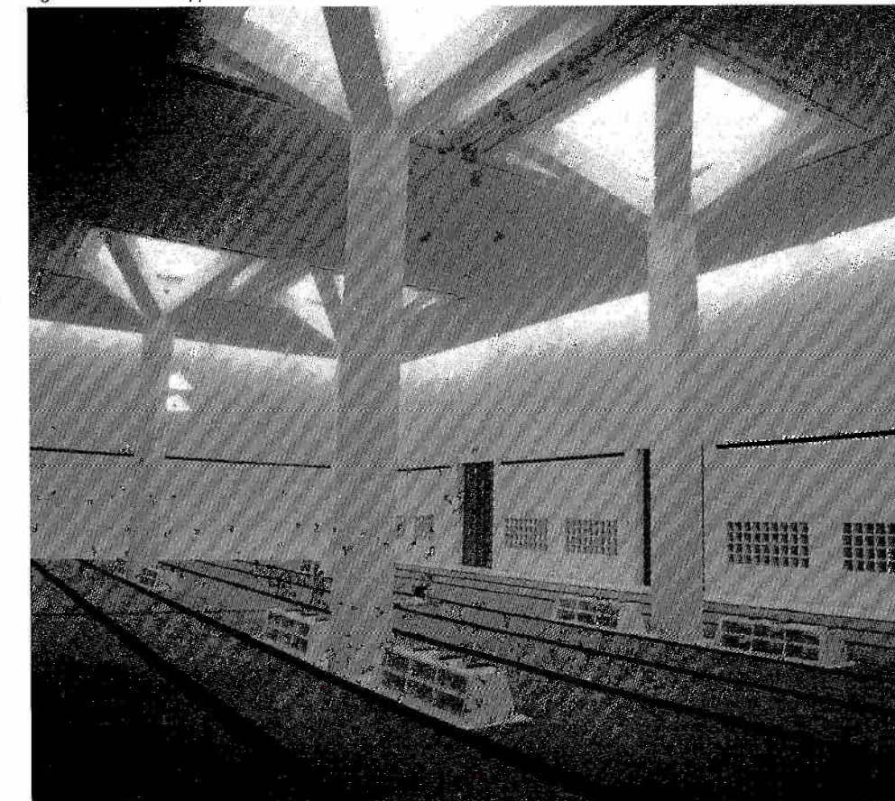
Fig 11.2 Internal support columns to roof
